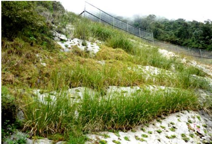
With these good results, the perfect interaction between Vetiver and the Eco Mortar was demonstrated in different soil conditions. The Eco mortar working on the steep slopes of hillside controlling surface erosion and water infiltrations and Vetiver System working from inside the soil giving strength and binding soils. More than 50.000 m<sup>2</sup> of eroded area has been recovered in a wide range of climatic conditions and different altitudes from sea levels to 2,800 m above sea level
